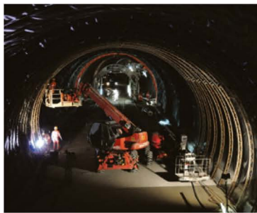
Tunnel de Court
